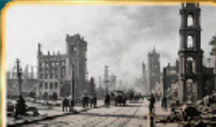
SAN FRANCISCO EARTHQUAKE 1906
