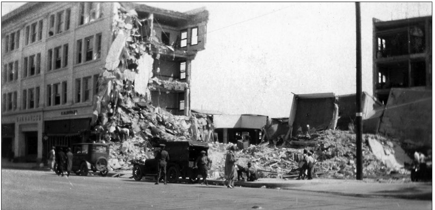
The corner of State and Anapamu with the remains of the San Marcos building and debris littering State Street.
