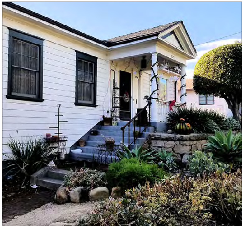
Exterior of 1821 Anacapa Street.
