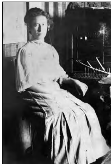
Marie York at switchboard
