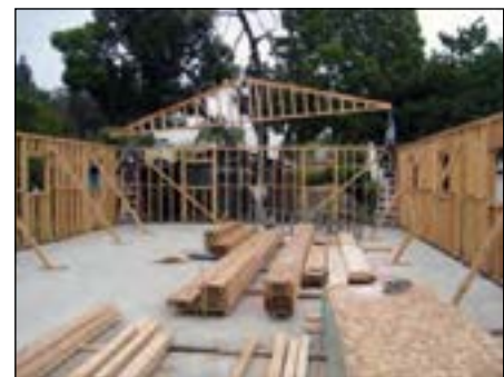
Framing stages of the library extension.
