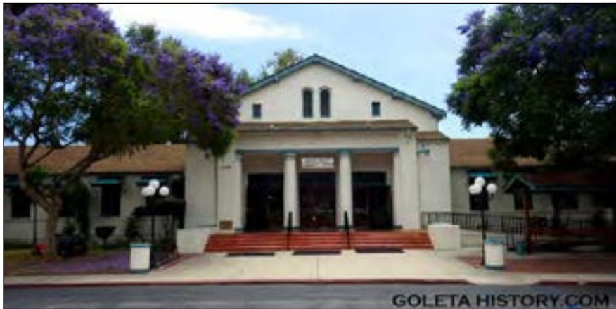
In 1979, a new home was at the Goleta Valley Community Center
