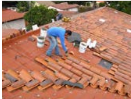
Installation of red tile roofing.
