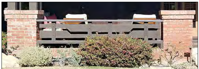
1920 Laguna Street porch railing. Credit: Betsy J. Green
