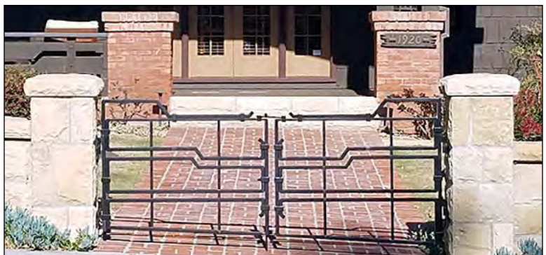
1920 Laguna Street front gate. Credit: Betsy J. Green
