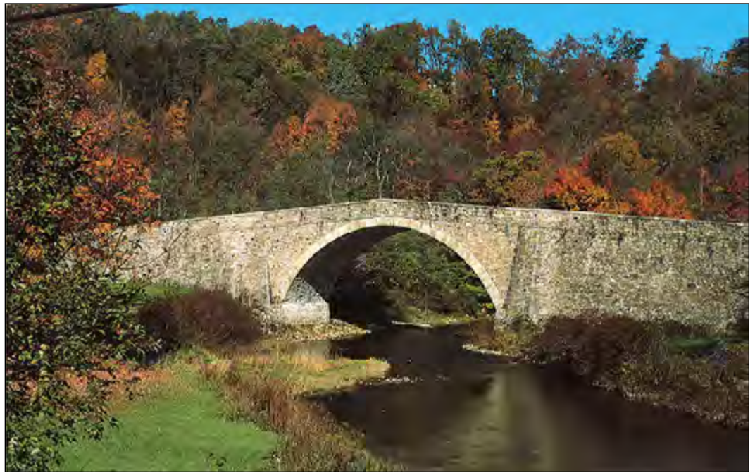
The Casselman River Bridge was constructed 1813-1814 near Grantsville, Maryland.
