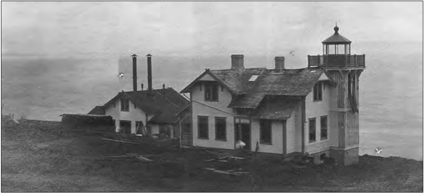
Point San Luis light station under construction. Rear of head keeper's dwelling and tower, rear of fog signal building.
