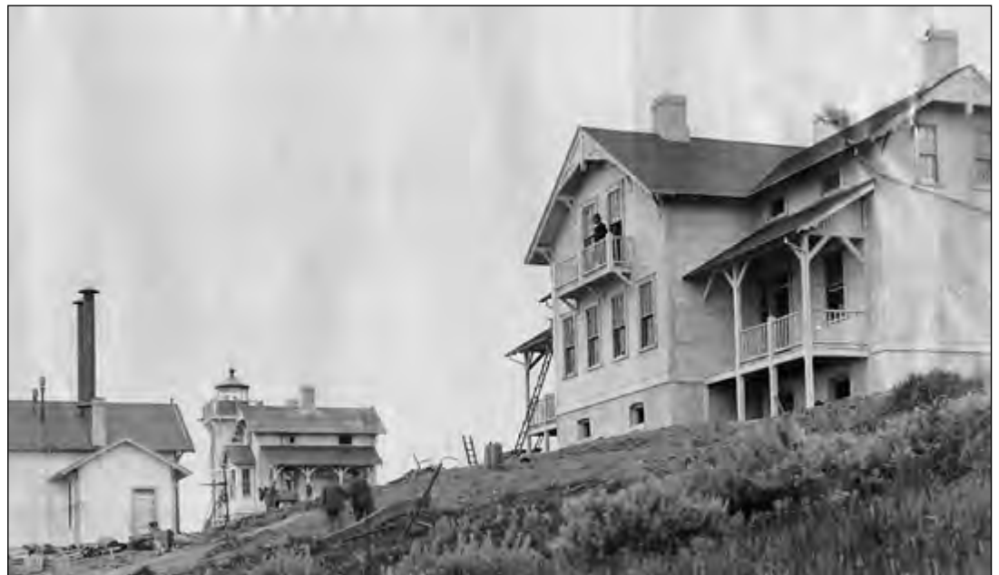
Point San Luis light station under construction. Double keepers' dwelling in foreground at right, fog signal building in foreground at left, head keeper's dwelling and tower in back.
