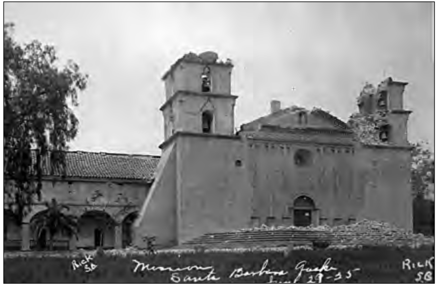
Damage to the Santa Barbara Mission following the earthquake of 1925.
