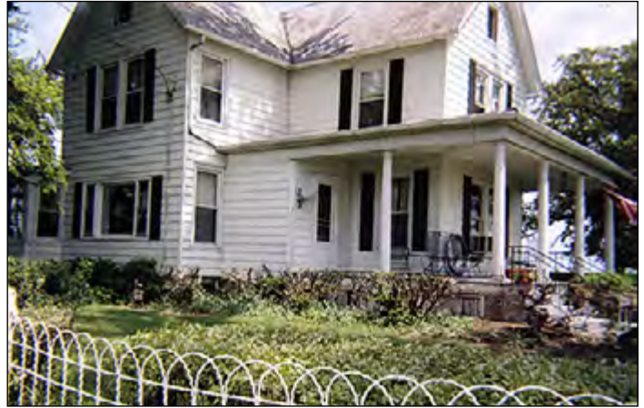
The farmhouse built by George Shute in 1908.
