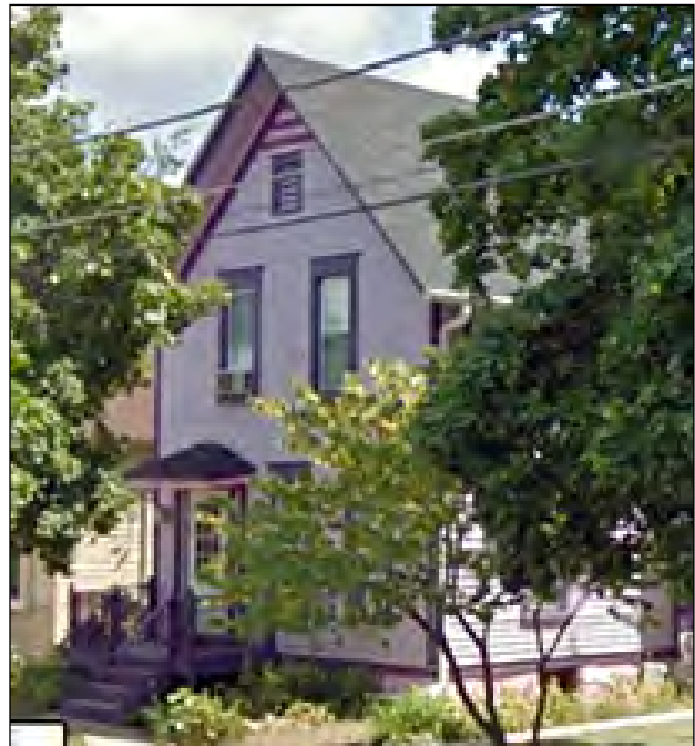
The little purple house in Elgin, Kane County, Illinois, that was owned by the Knickrehm family for 50 years between 1902 and 1952.
