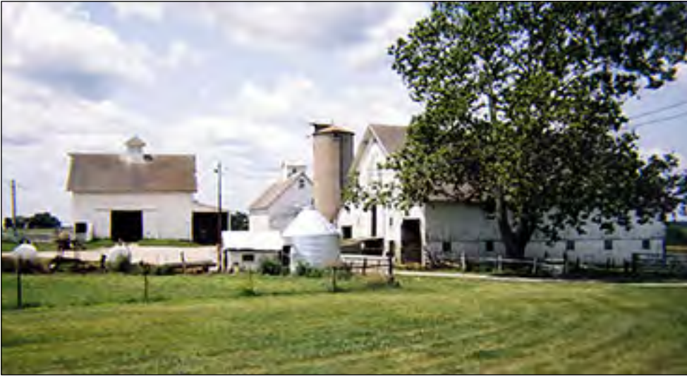
The farm buildings, including the original barn where my father and grandfather had left their names on the walls.
