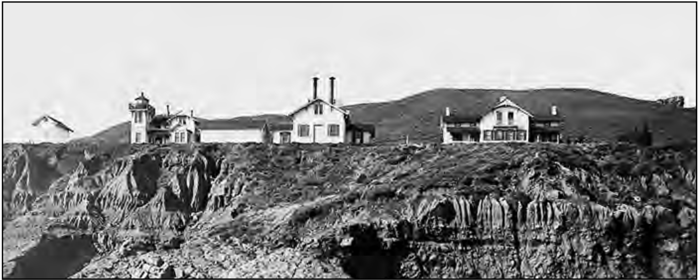
San Luis Obispo Light Station, California. Date: 2/22/1894 District: 18 National Archives Identifier: 45709181 Local Identifier: 26-LG-66-42 Container Identifier: 66 Creator: Department of Commerce. Bureau of Lighthouses. 1913-7/1/1939
