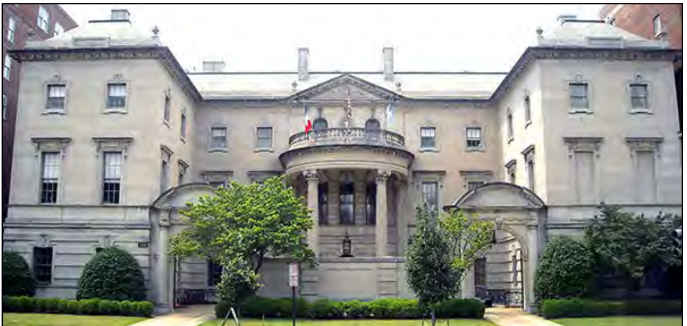
Andersen House, the home of Ambassador Larz Andersen that was bequeathed to the Society of the Cincinnati in 1937. 5
