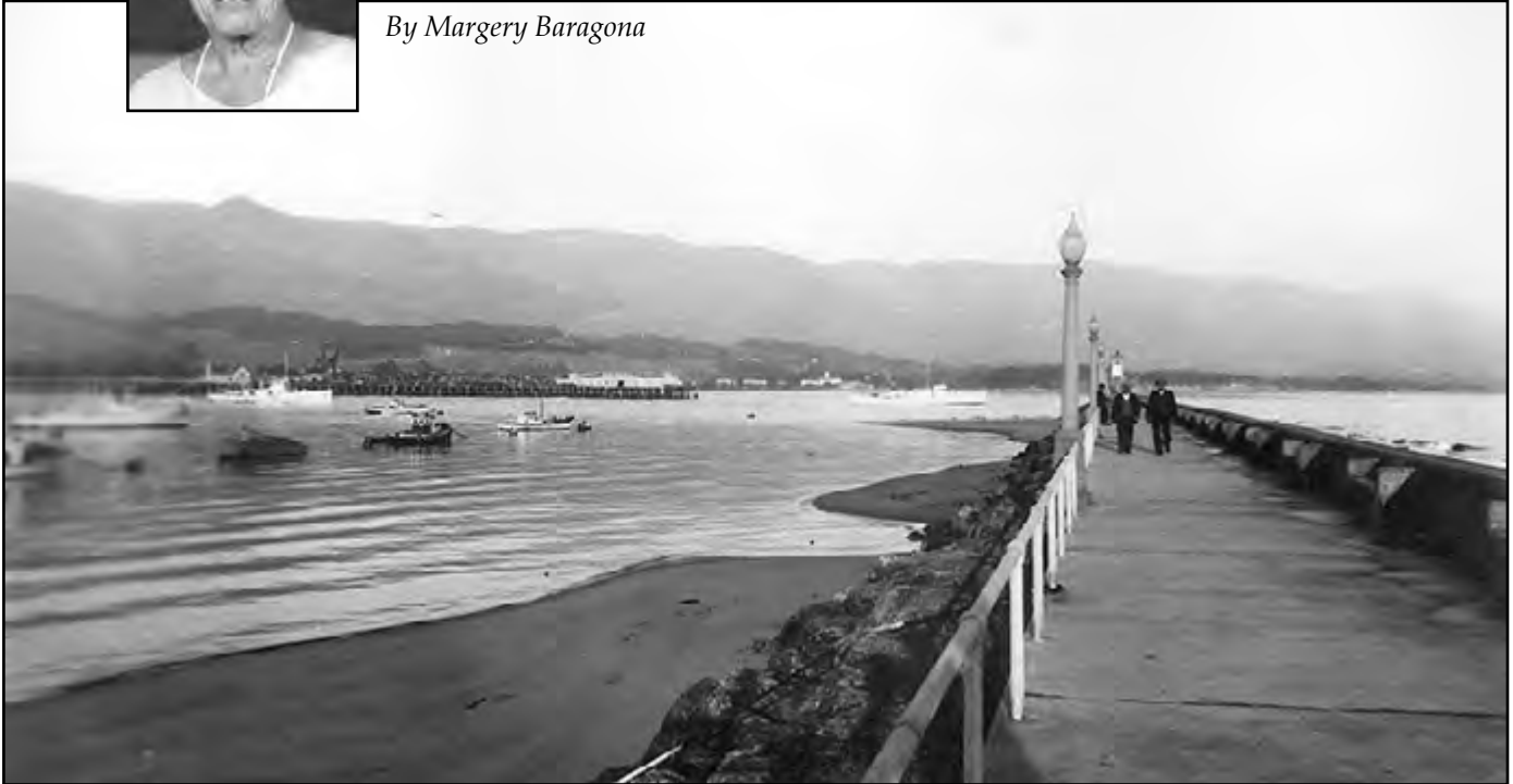
Santa Barbara Breakwater c. 1934, shortly after its construction. Photo from the National Archives and Records Administration NAID 295286.
