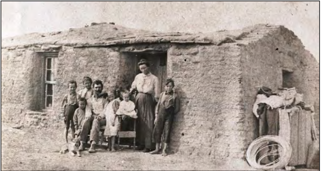
The Leroy Benshoof family in their new two-room sod shanty, built after the cyclone destroyed their first one.
