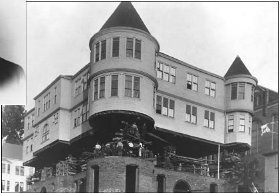
Building being moved by the Knickrehm Company in Los Angeles
