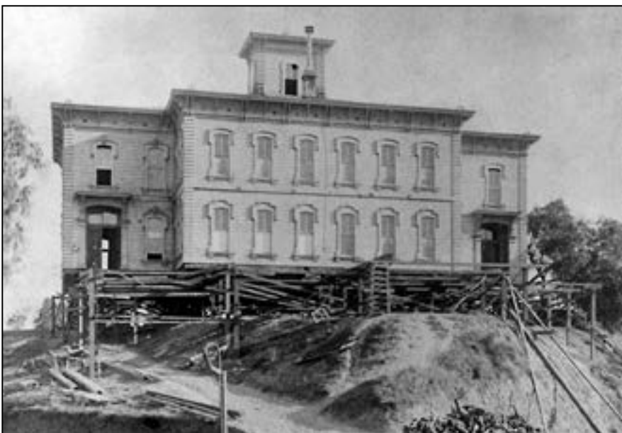
A building ready to move, Los Angeles, 1925
