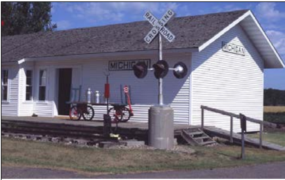
The Michigan Depot Today, Jim Wilson Photo
