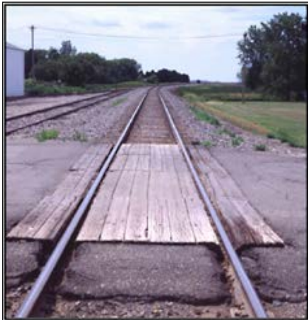
Looking West across First Street Collision Occurred at Curve in the Distance, Jim Wilson Collection
