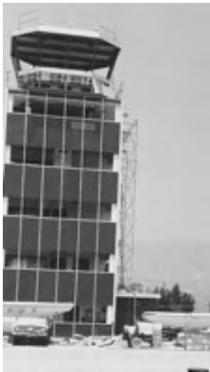
New aircraft traffic control tower construction Aug. 1962
