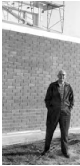
Bill checking out the construction site.
